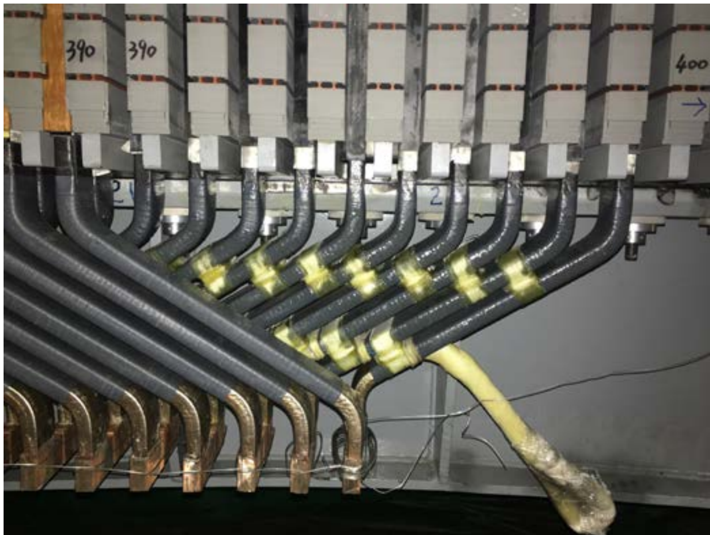
Figure 6: Karuma Generator Lap Winding
