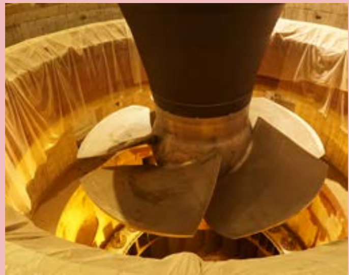
Lowering one of the Kaplan turbine units at Isimba HPP
