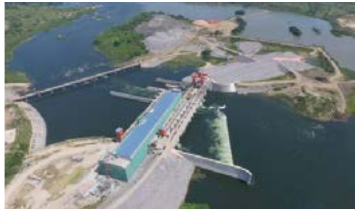
Aerial View of Isimba HPP after Second stage River Diversion
