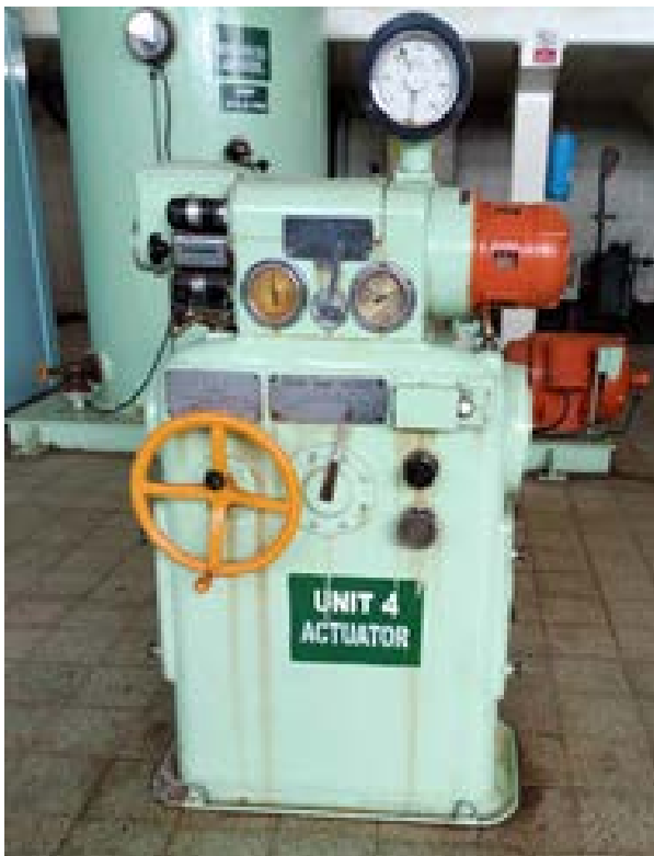
Figure 2: Actuator for the mechanical governors at Nalubale HPP
