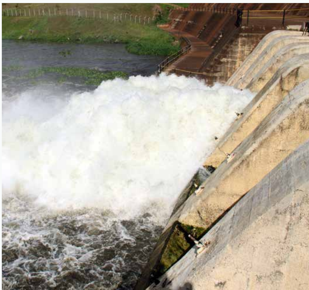
Spillway gates opened at Nalubaale Hydro- Power Plant
