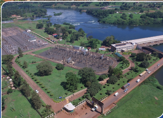
380MW Nalubaale-Kiira Hydro Power complex
