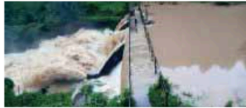
Muziba Small Hydropower Plant flooding in April 2020, attributed to reservoir silting
